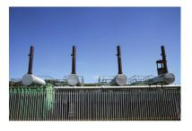
▲ Methane produced from rotting refuse is trapped and used for energy production to ease the energy crisis in California.
