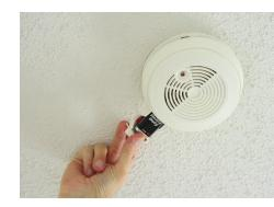
A Smoke detectors contain a small amount of americium-241. The  $\alpha$  particles emitted by this radioisotope ionize the air within the detector, causing it to conduct a tiny electric current. When smoke enters the chamber, conductivity drops and an alarm is triggered.
